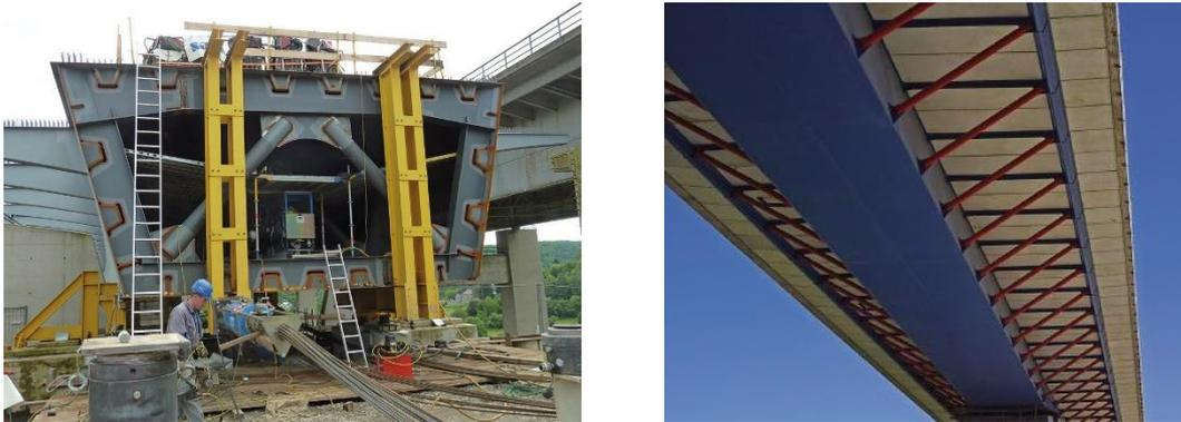
Figure 1: Design variants of tubular bracings inside or outside box girders: German bridges Heidingsfeld (left) [3] and Lennetal (right) [4]
