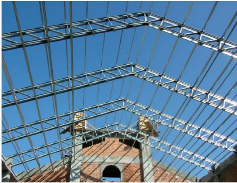
Figure 2.8: Roof trusses made of cold-formed steel-sections (Dubina et al., 2012) (p.40).
