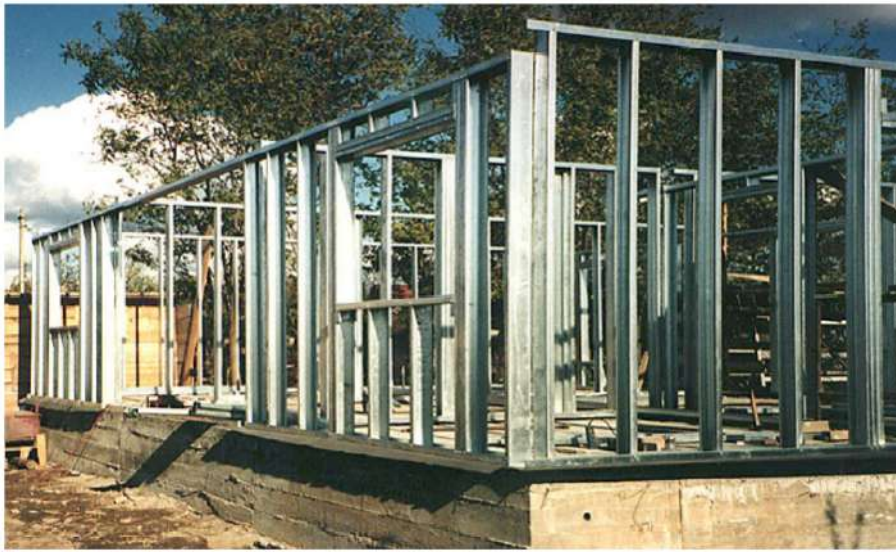
Figure 2.6: Wall partitioning made of cold-formed steel elements (Dubina et al., 2012) (p.36).
