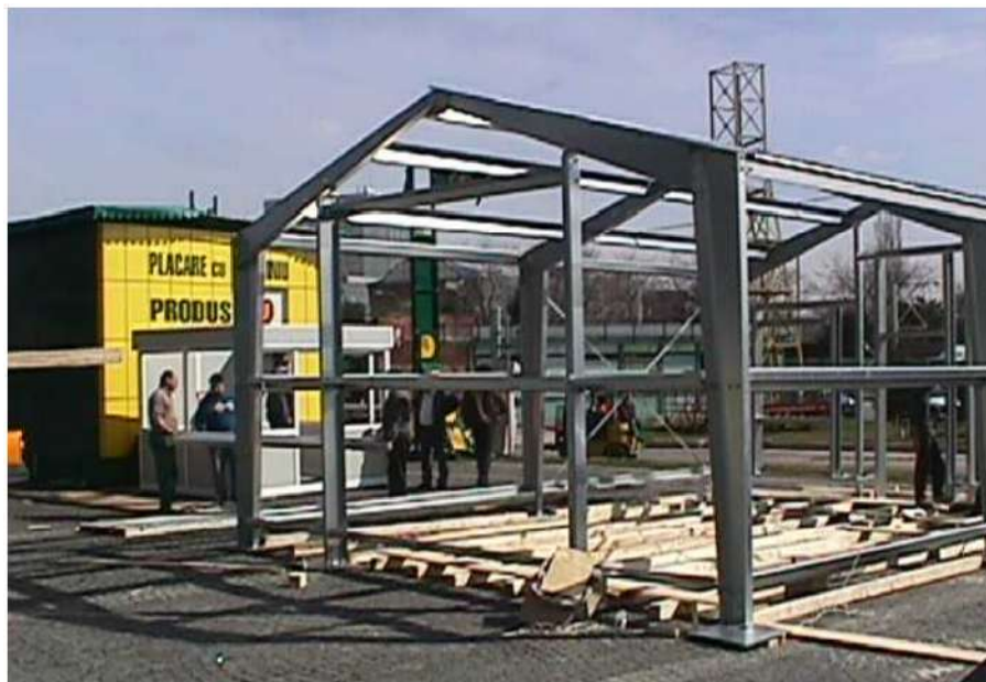
Figure 2.5: Steel framing made of cold-formed steel elements (Dubina et al., 2012) (p.35).
