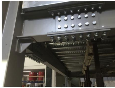
Figure 3-4 Position of stiffeners at the beam-column connection
