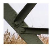
Figure 119 Single leg bolted connection
