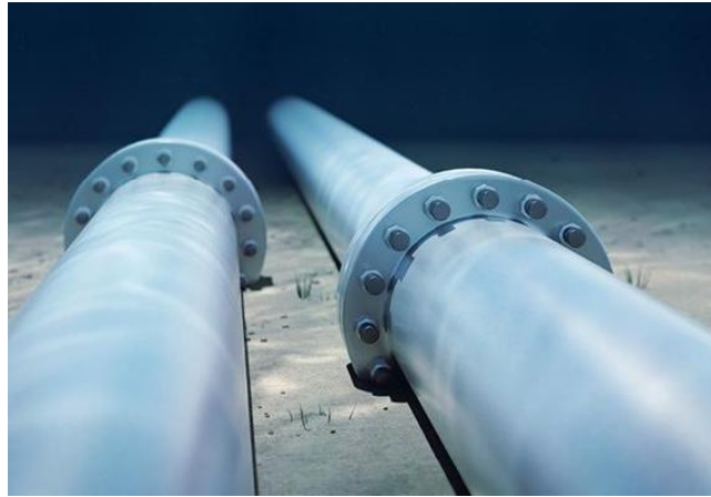
Figure 2.5: Underwater pipelines in the seabed with bolted flange connections [19]
