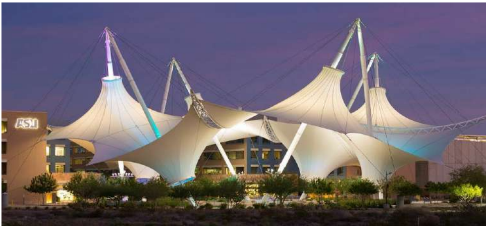
Figure 4: Skysong membrane roofing - tensioned structure at ASU University of Arizona [15]
