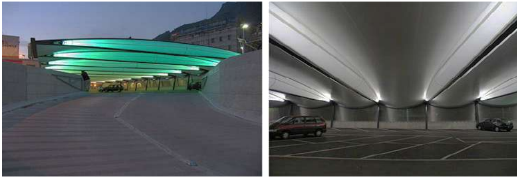
Figure 6: Tensairity carpark covering in Montreux, Switzerland [17]
