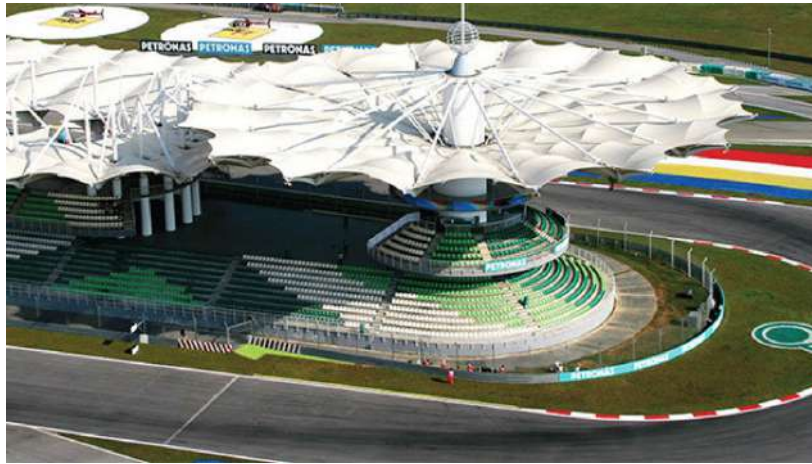
Figure 17: The space covering from above [27]
